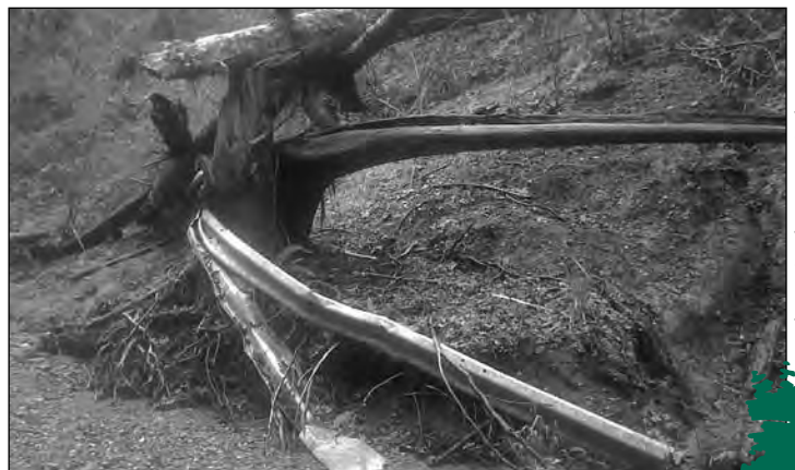
Illahee Road guardrail and large woody debris in Gilberton Creek.
