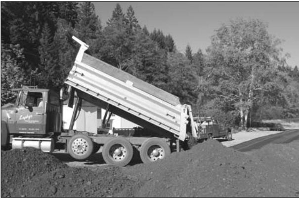
Klingel set-back dike under construction.
